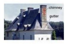
[countable] an open pipe fixed to the edge of a roof to collect and carry away rainwater
